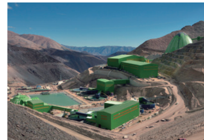
Caserones Copper Mine
