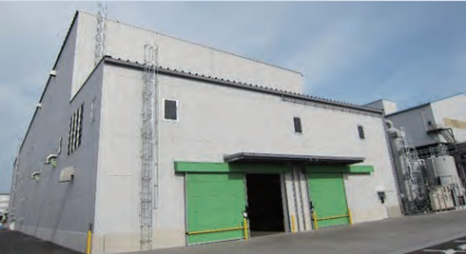
New nickel powder plant at Wakamatsu Plant
